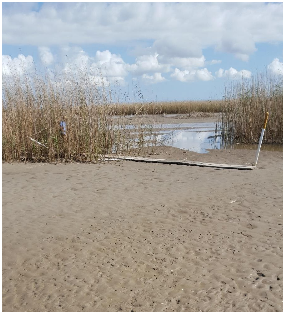
Figure 51b. Photograph of the boardwalk at CRMS2627 buried in sediment in September, 2016. Boardwalk was constructed 1.5' above the marsh surface in 2008.
